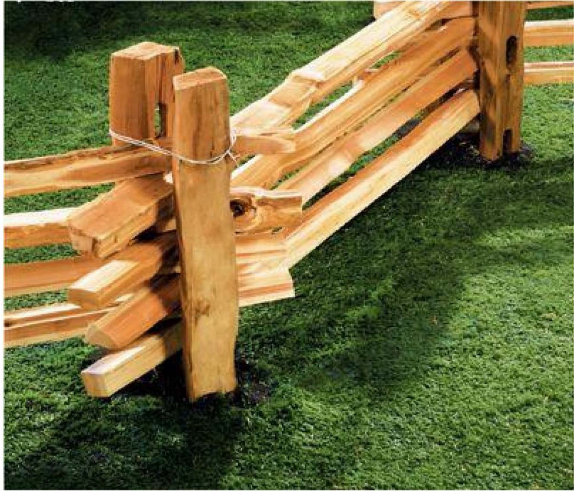
The Virginia Rail Fence exhibits a very familiar style to anyone who has spent much time in countryside that was cleared and farmed in the 18th and 19th centuries. Since nails were scarce, these zigzagging post- and-rail fences were popular because they are held together with only wire or rope.
