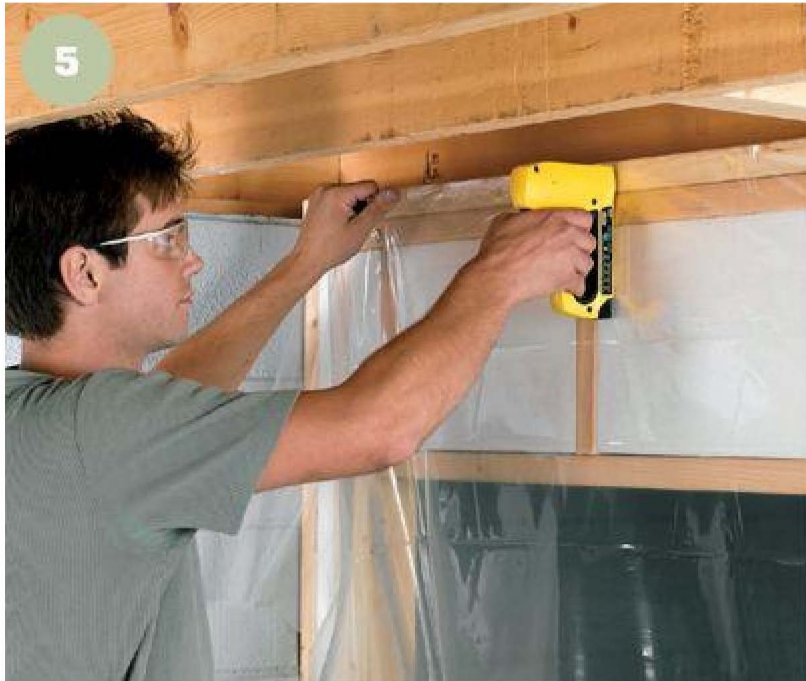
5 Staple a sheet-plastic vapor barrier to the basement side of the walls where condensation is likely to form.
