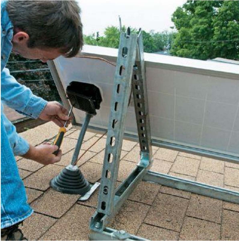
Connections for the feed wires that carry current from the collector are made inside an electrical box mounted on the back of the collector panel.
