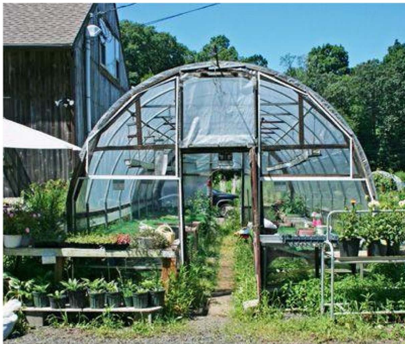
Hoophouse frames can be made from wood instead of PVC plastic. Wood allows you to attach plastic sheeting with retainer strips and staples.
